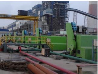
MACMET has been supplying water screening equipment to Steel, Power, Oil and Desalination Plants, both in India and Overseas for several decades. Coarse, medium and fine screening equipment are used in effective combination to remove debris, weeds, branches, grass, fish, etc. from water sourced from rivers, lakes and oceans.
